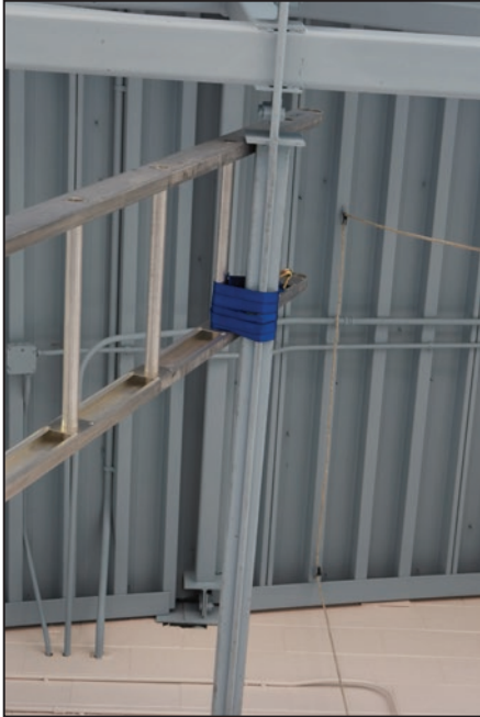
Figure 10c: Close up of the 24' anchor point
